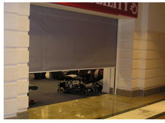
**The roller unit** incorporates a motor, planetary gearbox, and control electronics with a microprocessor. The microprocessor monitors the resting position when rolled up and independently regulates the closing speed to a maximum of 0,15 m/s (6in / sec).
