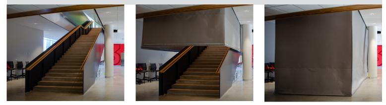
3 Passive smoke containment by Installing a motorized smoke curtain on the 4th floor to isolate one side of the atrium
