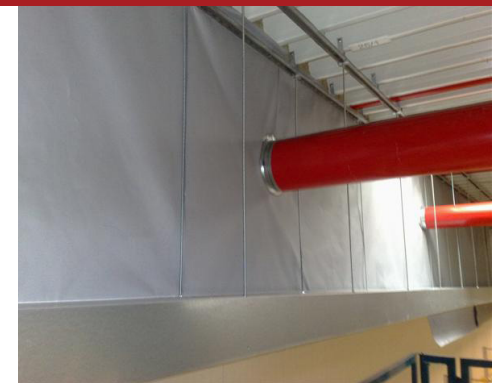
Its prefabricated metal sleeves allow penetrations to be made in various sizes and shapes.
