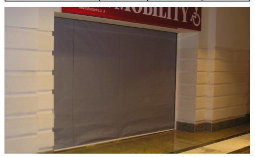
A bottom bar is attached to the bottom of the curtain and serves to ensure that the curtain operates as designed and also that it remains stable when unrolling.
