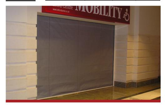
A bottom bar is attached to the bottom of the curtain and serves to ensure that the curtain operates as designed and also that it remains stable when unrolling.
