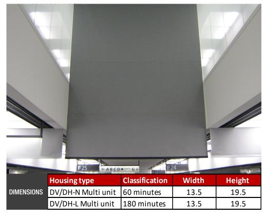
A bottom bar is attached to the bottom of the curtain and serves to ensure that the curtain operates as designed and also that it remains stable when unrolling.
