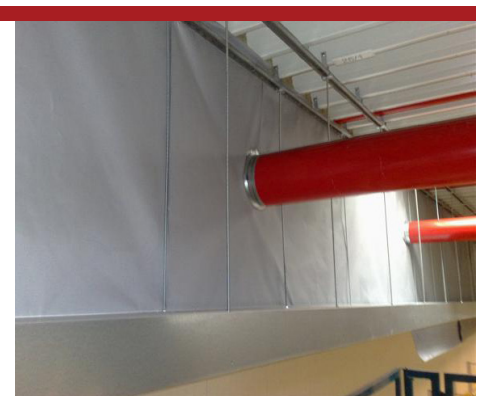
Its prefabricated metal sleeves allow penetrations to be made in various sizes and shapes.
