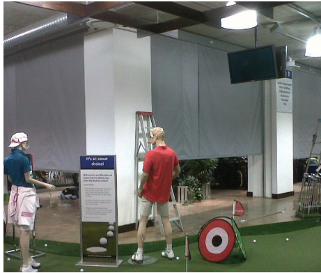
Retail - fire curtain in mid position
